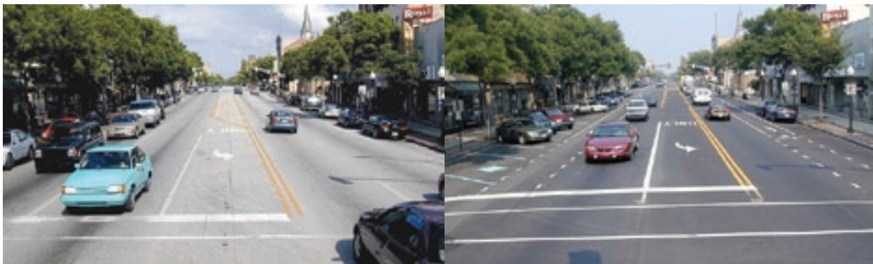
In a complete streets project in historic downtown Pottstown, Pa., a lane each way was removed, and a center lane, more (angled) parking and bike lanes were added.
