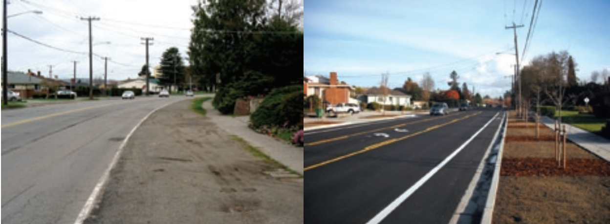
An example of a complete streets project from S. Columbian Way in Seattle, courtesy of the Seattle Department of Transportation. A street with an inadequate sidewalk, lanes that were too wide and no safe place to bike received curbs, sidewalks, narrower lanes, and a curb bike lane. Complete streets policies ensure that new roads and refurbished roads account for the needs of all users.
